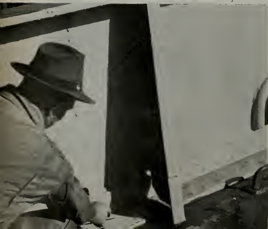
Closeup view of riveted gunwale angle installation on SS Abigail Adams.
